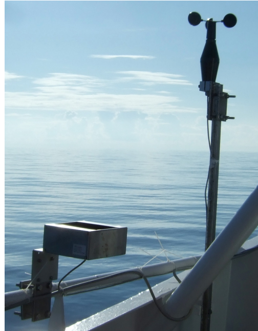
Fig.11.1 Optical disdrometer, anemometer and rain sensor installed on deck.
